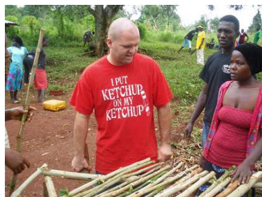
Building a sun drying stand in the compound
